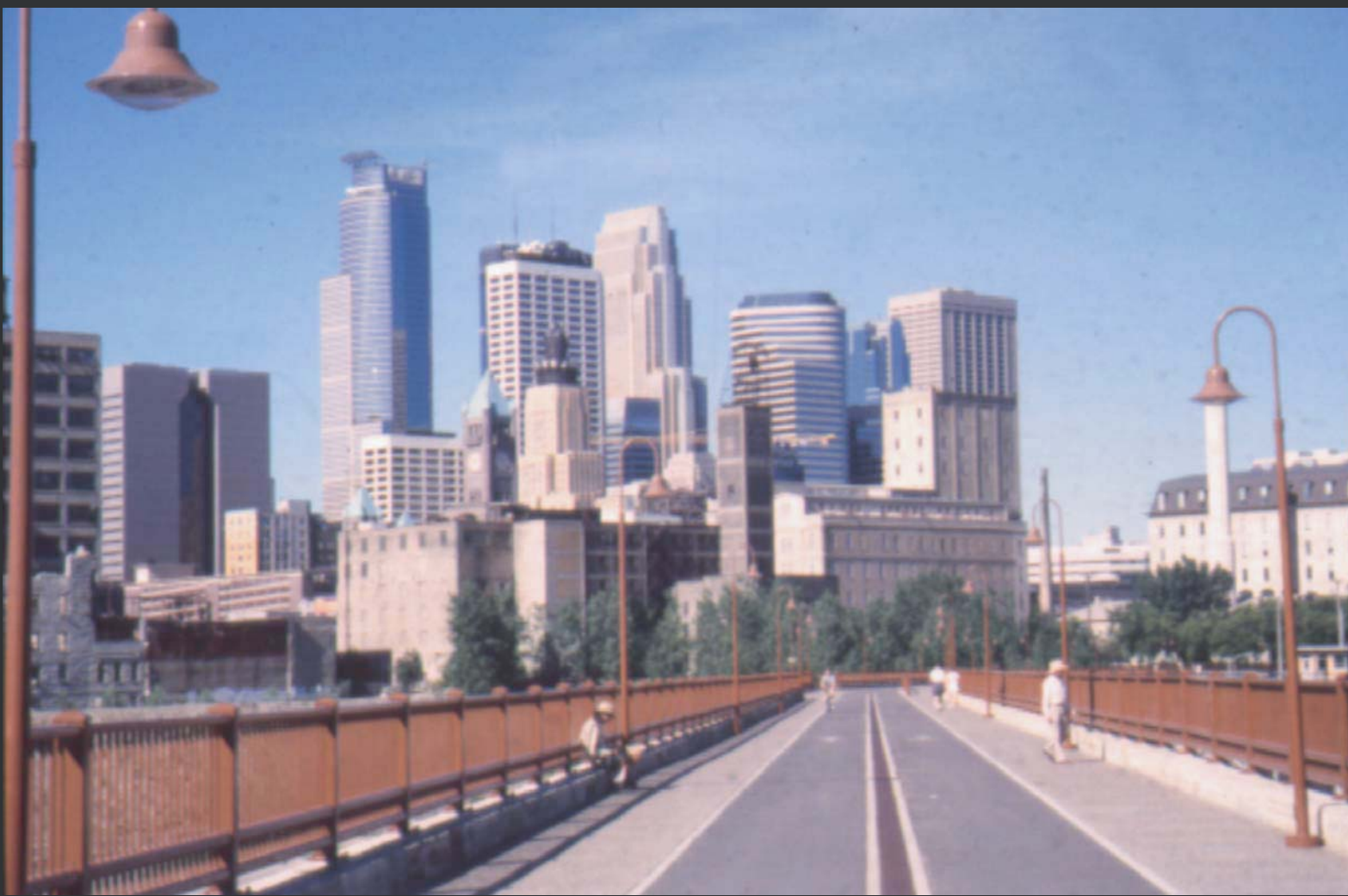
Stone Arch Bridge - Minneapolis, MN Designed by A.G. Lichtenstein & Associates, Inc.
