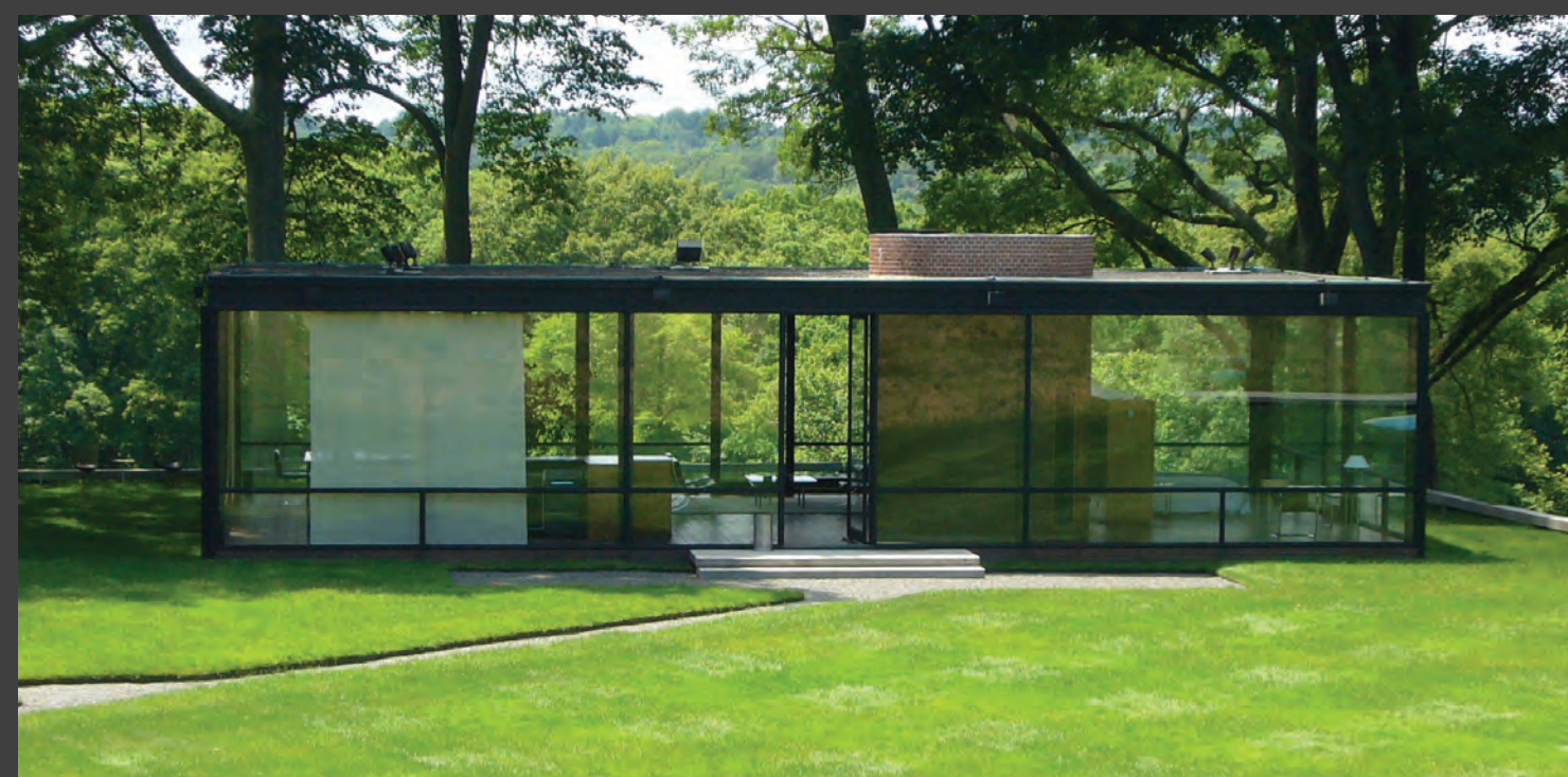
Glass House by Philip Johnson. Built in Connecticut in 1949, the house has a bold emphasis on exposure to the landscape from within its glass walls.
