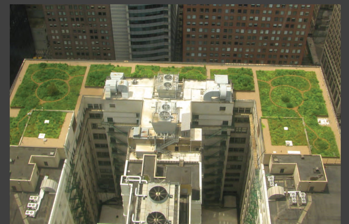
The extensive green roof on Chicago's City Hall. Designed by William McDonough and completed in 2001.
