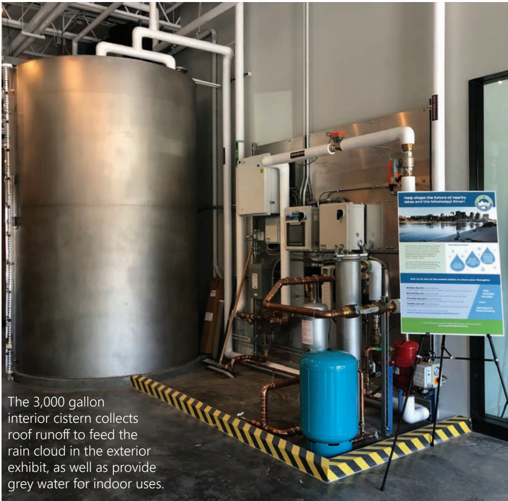
4. Interactive Exhibit: roofwater harvesting system with mechanicals exposed for education (left) is the water source for the pocket park exhibit (right)
