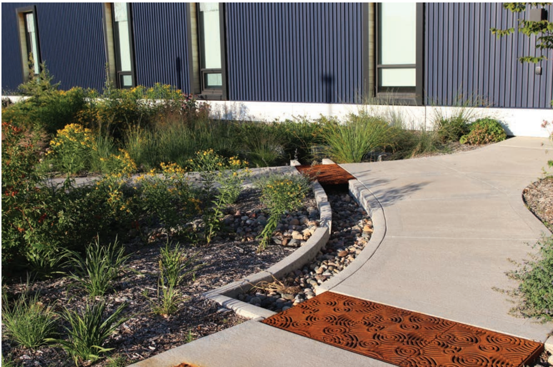
13. Secondary Entry Runoff Conveyance: from workshop roof to bioretention rain gardens at outdoor classroom
