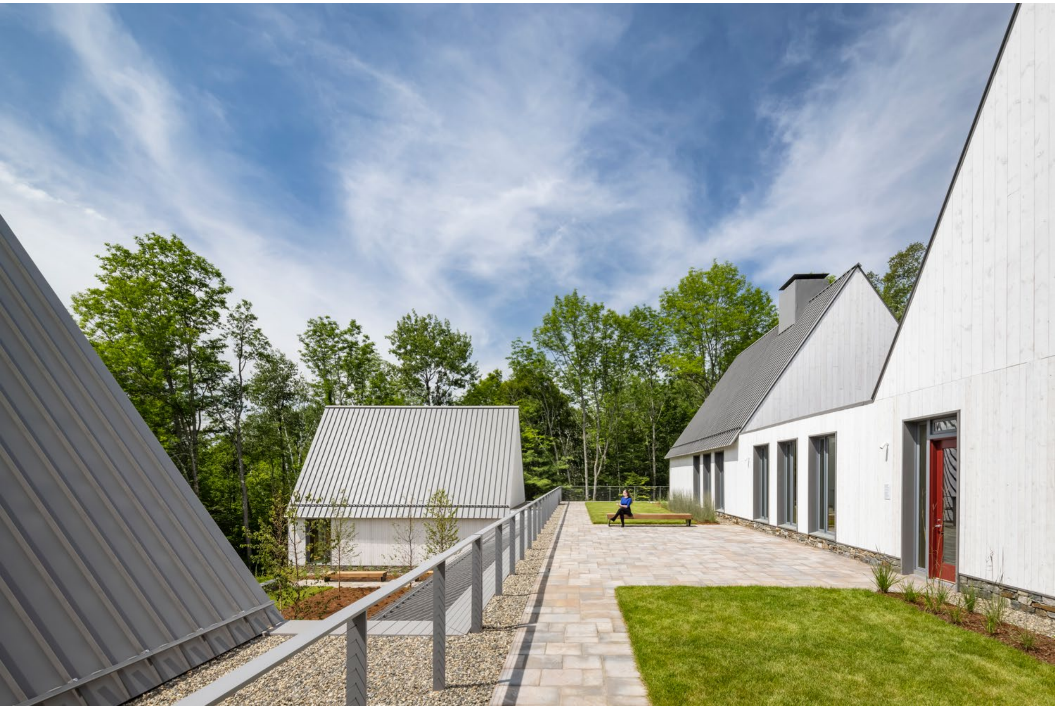
UPPER TERRACE GREEN ROOF | To foster a connection to the outdoors, the green roof terrace sets a stage for events and casual interactions where musicians can practice together in the open air, eat meals, or have happy-hour gatherings all while taking in views of the surrounding picturesque Green Mountain landscape.
