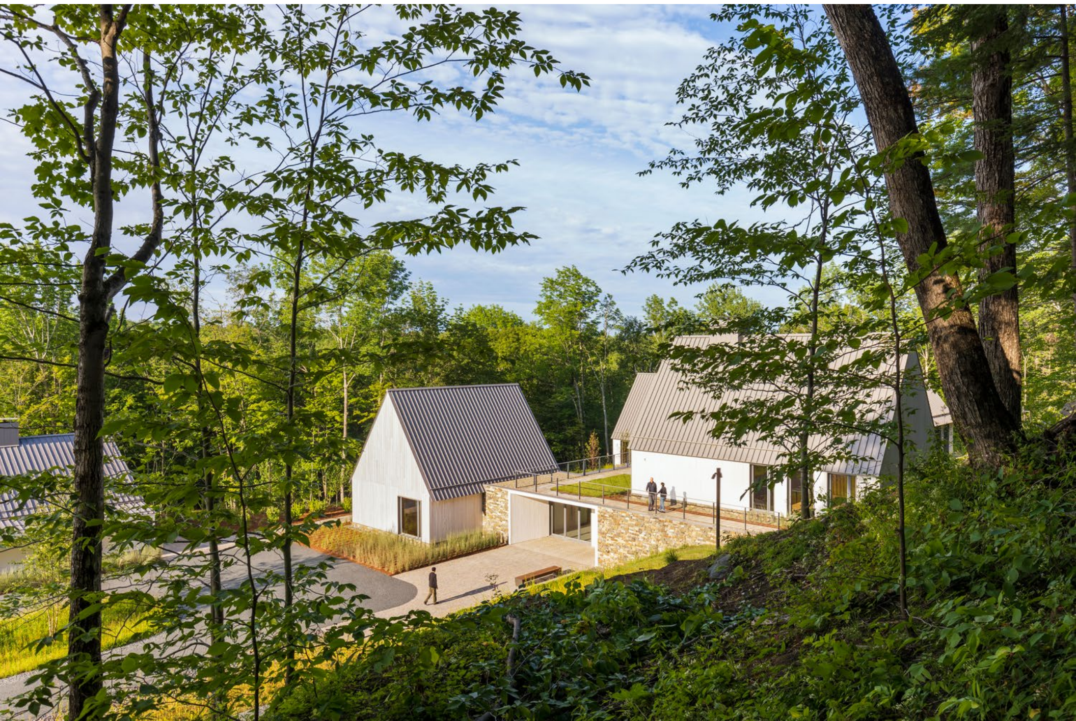
GREEN MOUNTAIN TERRAIN | Ledge rock and mountainous terrain played a significant role in the project. Planting selection for erosion control, infiltration capacity of the subsurface condition for storm water management, the ability to plant new trees, earthwork for foundations, all required design consideration and close communication of on-site conditions during construction.
