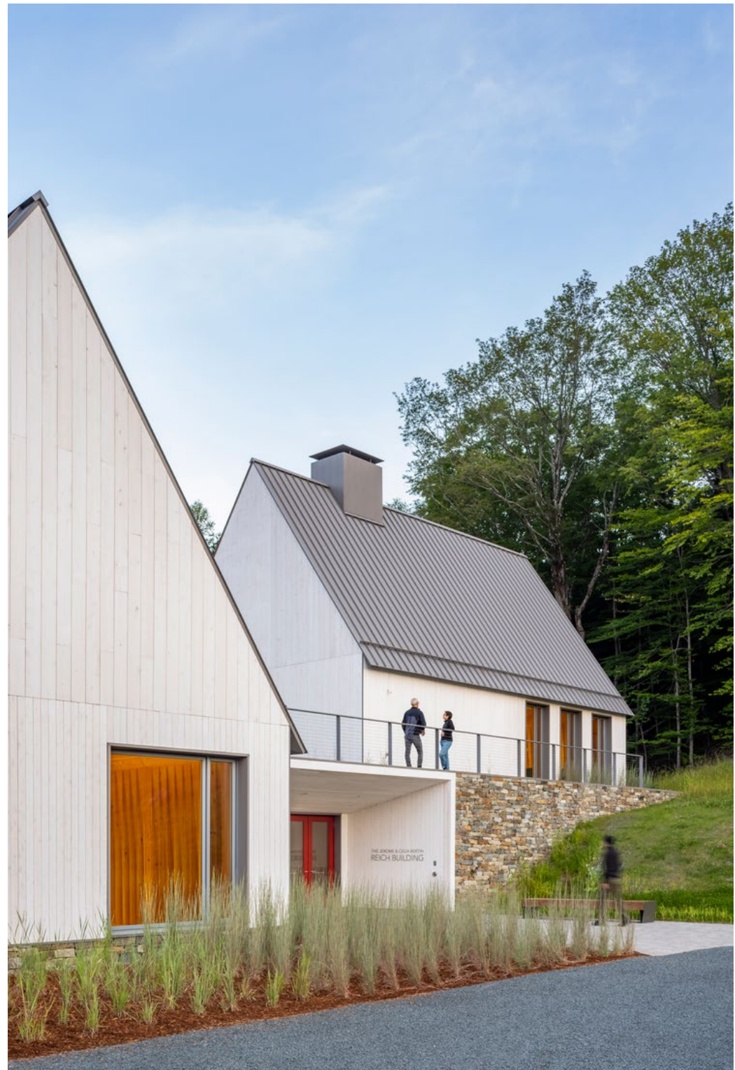
LOWER LEVEL ENTRY
