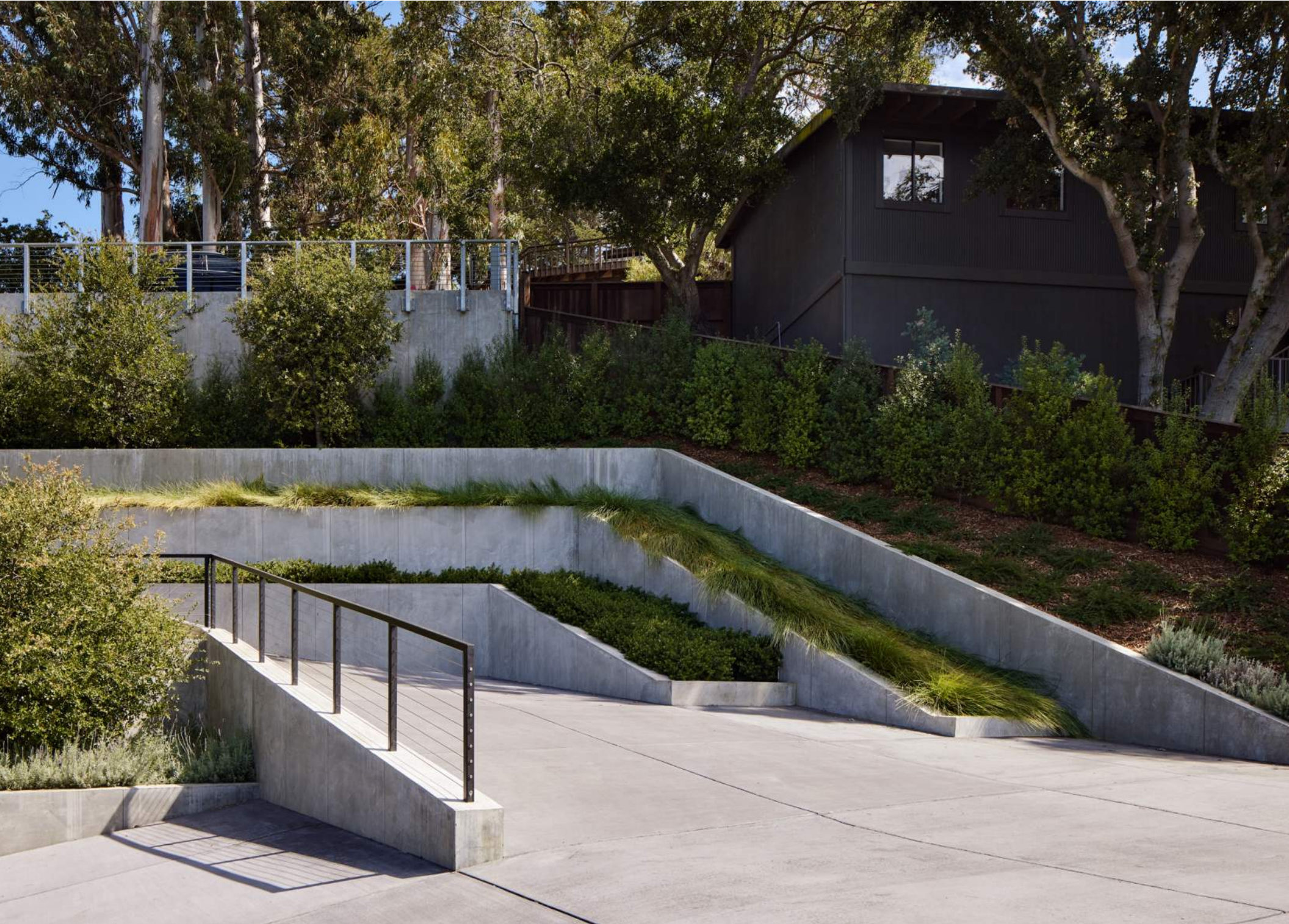
The interplay of concrete paving, site walls, railings, and textural plantings create a simple but dramatic entry sequence. The retaining walls, a necessary requirement, do not read as such; rather they create an artful sculpting of the site topography.
