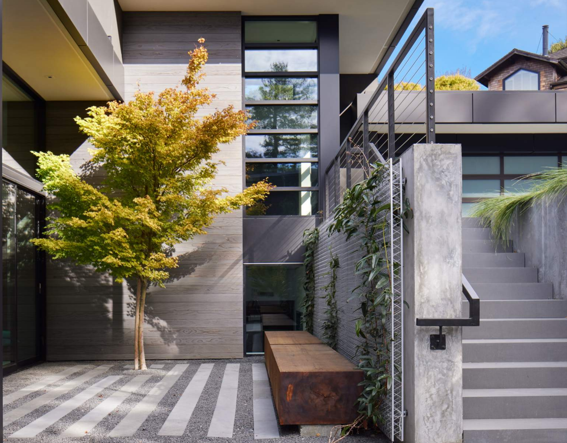
The entry stairs and courtyard, featuring stone detailing and a bench fabricated of wood salvaged from a tree removed prior to construction.
