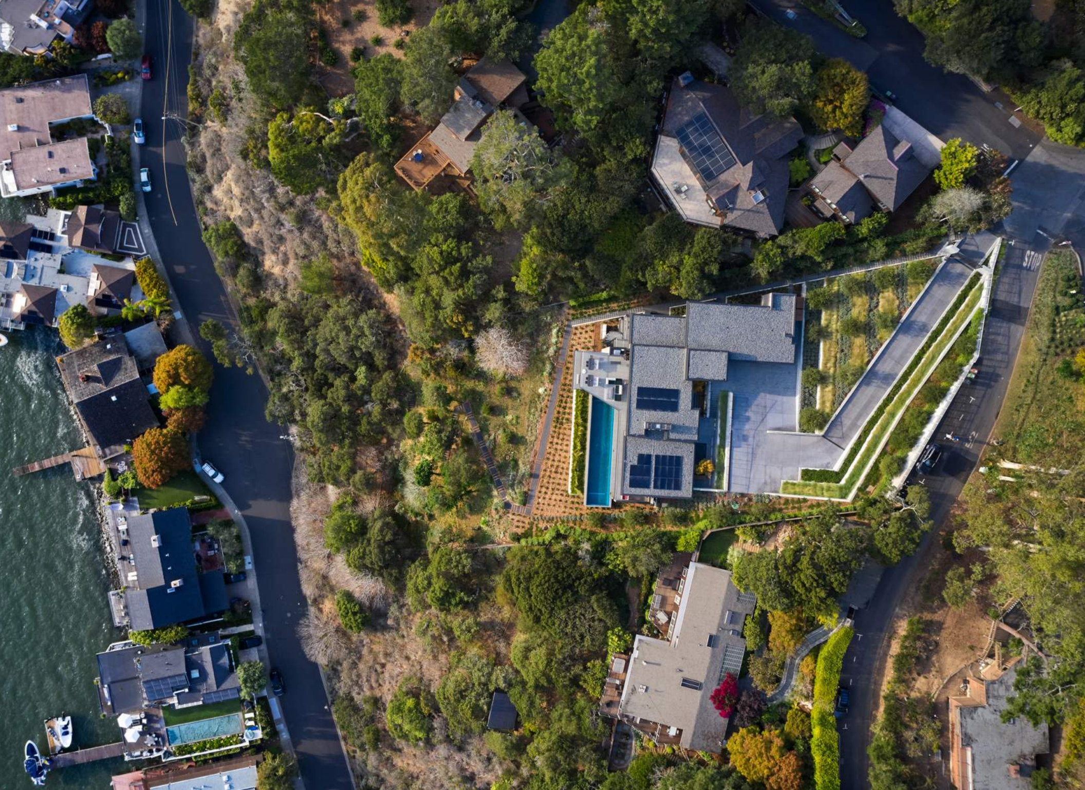
Bird's eye photograph illustrating the strong geometry of the upper entry garden and the related, yet less structured, landscape of the meadow and grove hillside.
